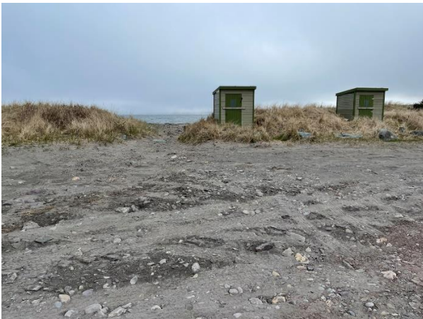
Figure 11: inundation of the toilets by sand and sediment.
