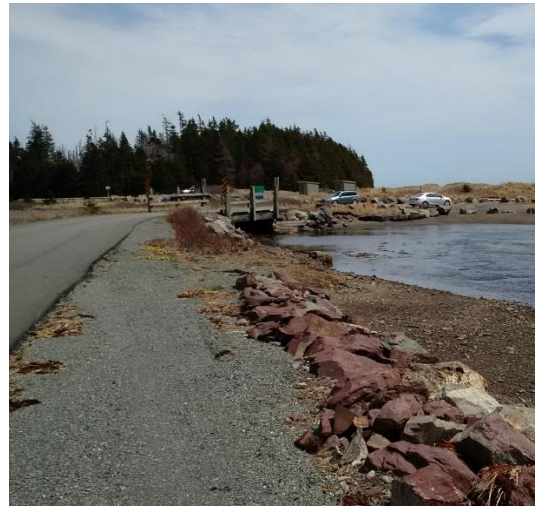
Figure 9: Pondville South Road and bridge.
